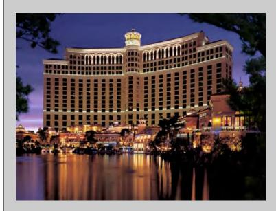
The Bellagio Hotel and Casino in Las Vegas has an EIFS skin or exterior cladding. This material works well in cities with extremely dry climates. For disposable structures, structures not intended to last for more than 50 years, EIFS is a good cost saving measure.
