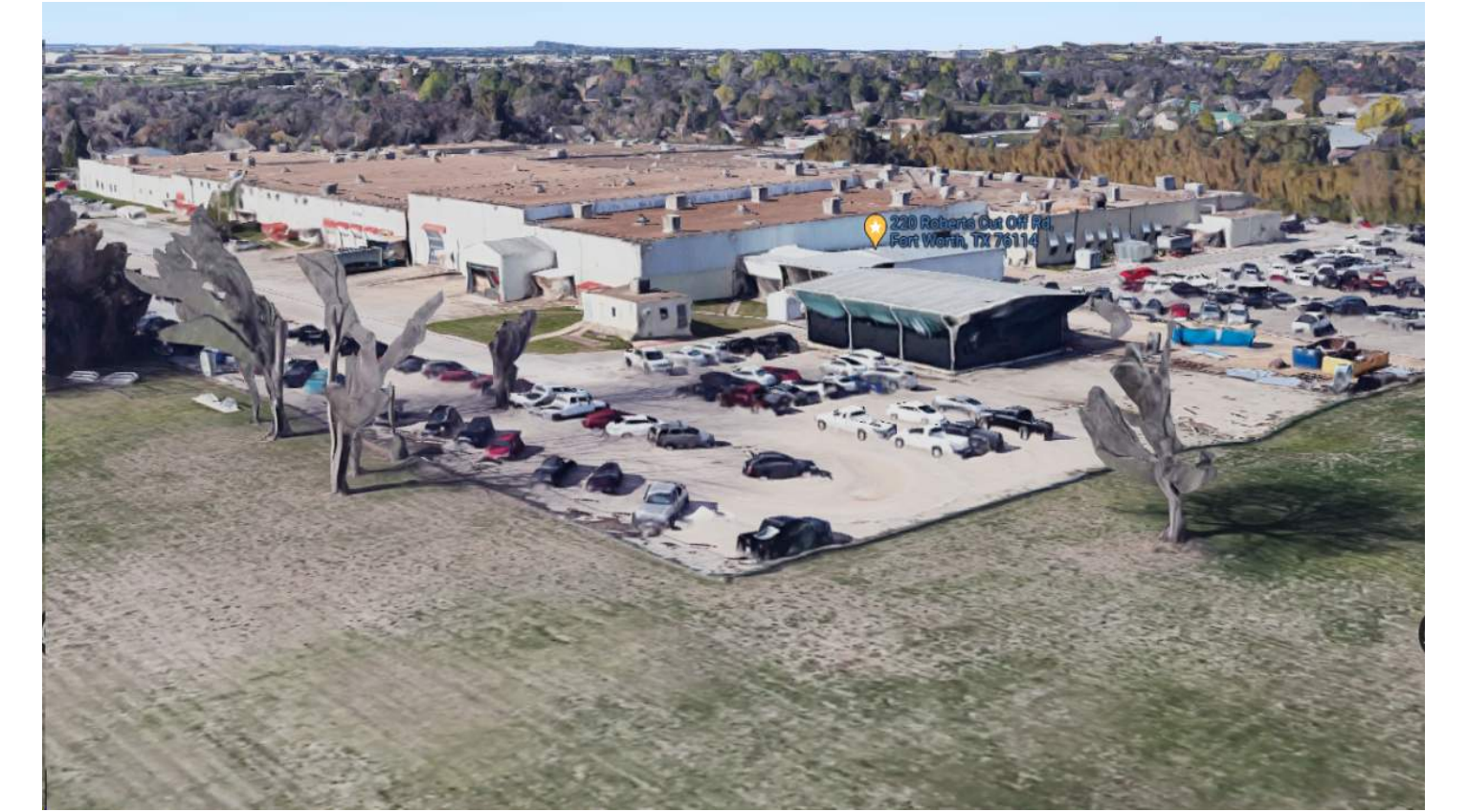
VIEW FROM SE BEFORE
