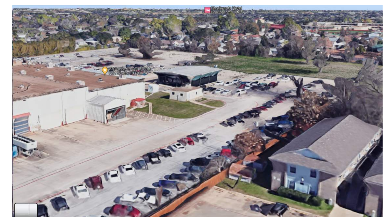
VIEW FROM SW BEFORE
