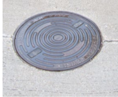
Existing Manhole Cover
