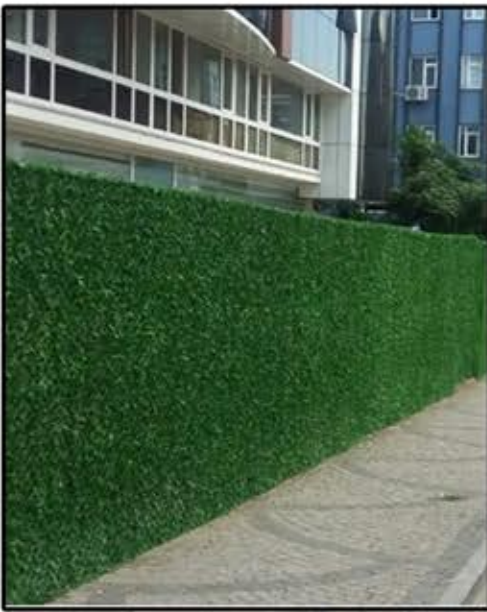
8" CHAIN LINK GREEN FENCE
