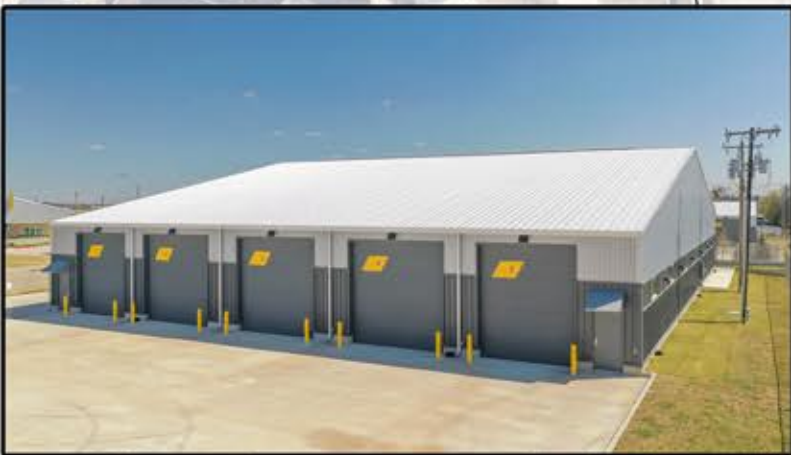
GRADE LEVEL DOORS
