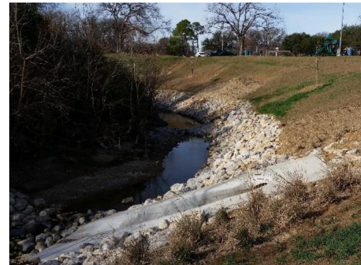
Sandy Lane erosion control before & after
