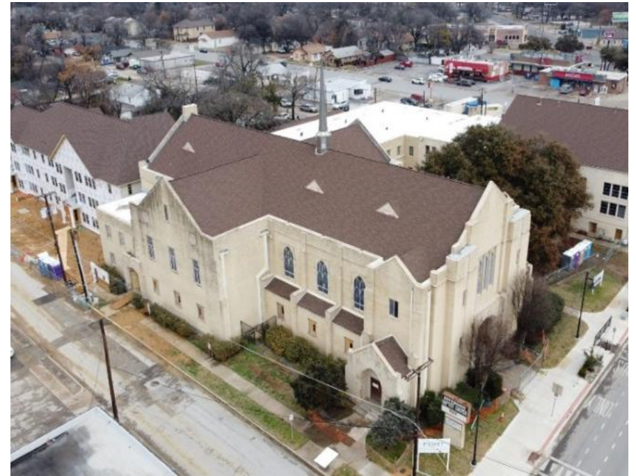
Preservation staff worked with developer of Cielo Place on Race Street to save the main sanctuary, integrating it into new senior-living development
