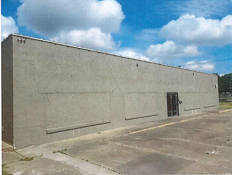
Figure 5 - 120 Riverside facing Riverside – existing shoddy masonry repairs, etc. are show cased in this photo
