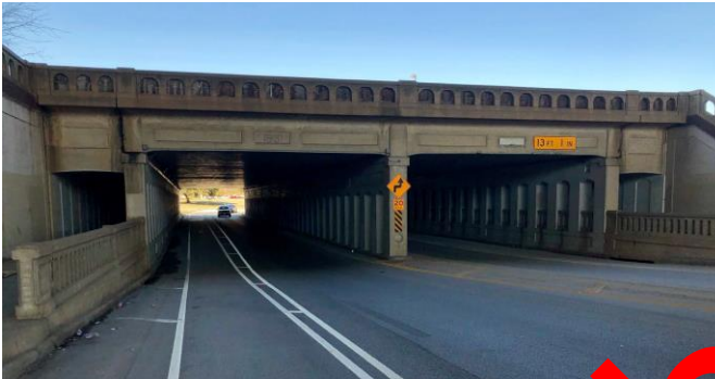
SOUTH MAIN TUNNEL
