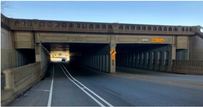
SOUTH MAIN TUNNEL
