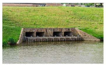
**Figure 6-14.** This TRWD trash basket traps debris and allows water to pass through, photo by City of Fort Worth.
