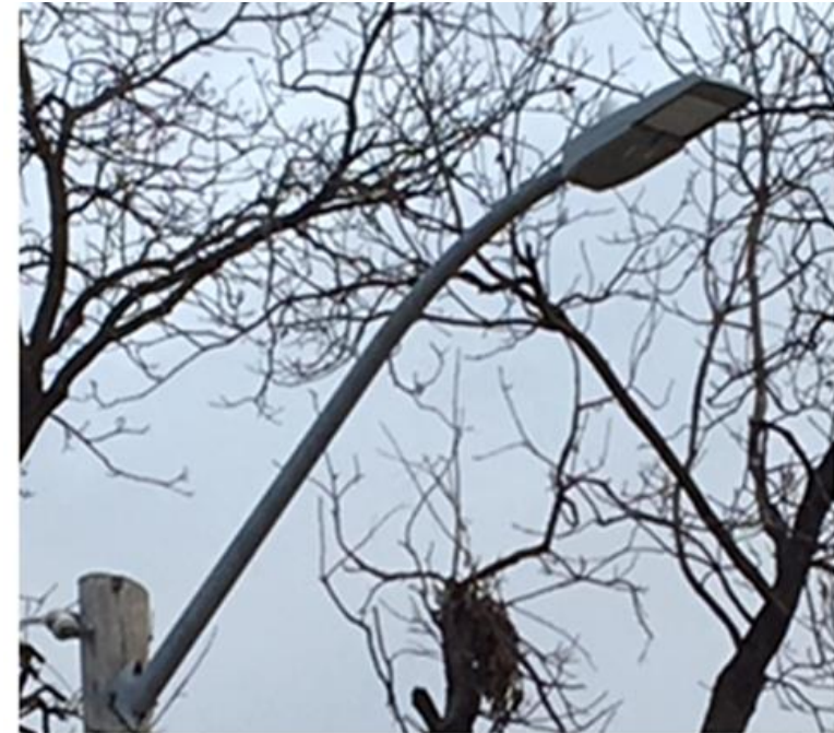
Wood Utility Pole with NEW LED
