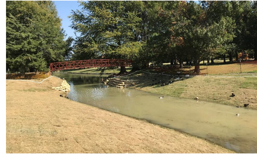
Candleridge Park – Erosion Control
