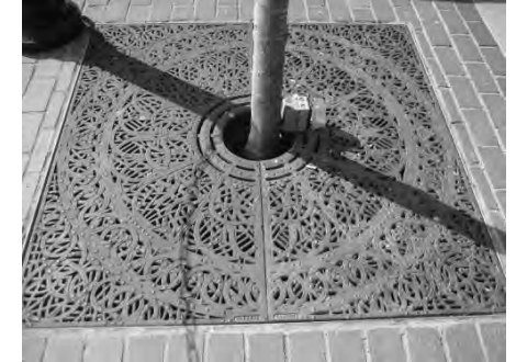
Tree grates provide space for the tree while allowing pedestrian traffic
