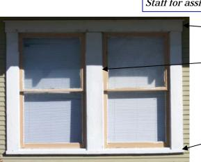
Always double the width of trim between paired windows. Make sure to include a wood drip cap above the trim and a wood sill. Drip caps help to prevent water from seeping behind the window unit and prevent water damage to the wall.
