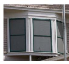
Solar screening is more opaque than traditional screening. This allows for more privacy while still allowing for air circulation. It will reduce the amount of light infiltration, by reflecting the sun's rays and because of its thickness it will help to trap heat in the winter months. The reflection of the sun ray's will also extend the life of your window unit.
