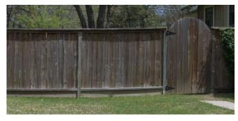
LEFT: It is preferable for wood privacy fences to be capped. The wood cap helps to shed water, increasing the longevity of the fence.
