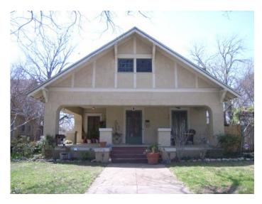
LEFT: The half timbering in the front gable of this structure identifies it as an Arts and Crafts structure, but it also serves as expansion and ventilation joints for the stucco veneer.
