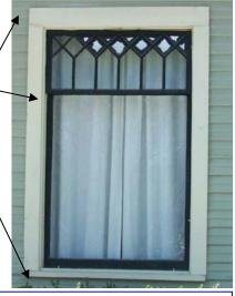
If a wood window is deemed non-repairable give special attention when choosing a replacement. Consider material, size, grid pattern and installations. Material changes MUST be approved by the HCLC but are generally not approved. Replacement windows should be recessed mounted, meaning they are not flush with the exterior of the wall and fit the original opening. Often the dimensions are difficult to replicate, ask Staff for assistance.
