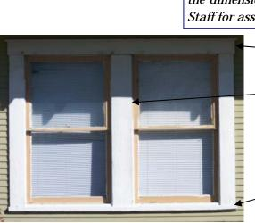
Always double the width of trim between paired windows. Make sure to include a wood drip cap above the trim and a wood sill. Drip caps help to prevent water from seeping behind the window unit and prevent water damage to the wall.
