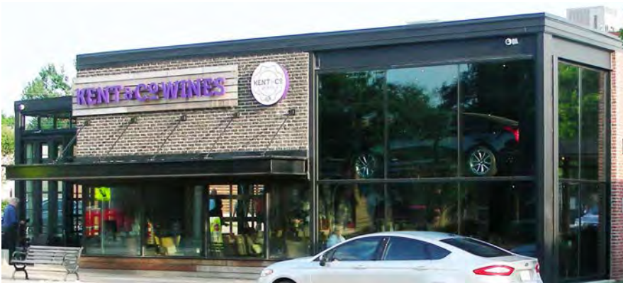
» Street level activation (shopfront)
