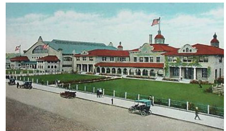
The Coliseum and Exchange Buildings sit side by side on the north side of Exchange Avenue. A green lawn and rail fence are key features.
