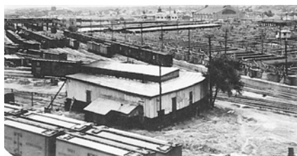
Rail spurs wound through the packing plants, allowing loading of final products onto rail cars.
