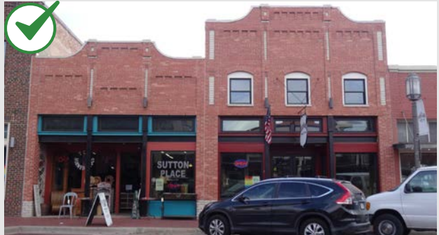
After: rehabilitation of historic building with reconstructed cornice, new windows and simplified interpretation of historic storefronts.
