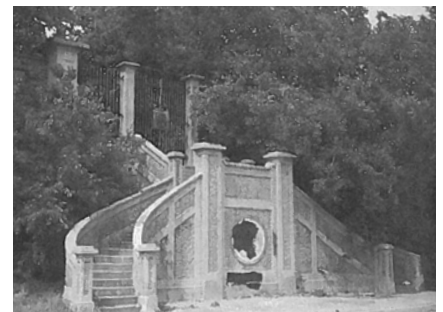
The historic Swift & Co. stairway once served as the south entrance to the Swift complex. This stairway still stands along 23rd Street and is landmarked.
