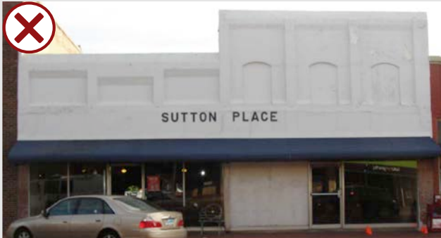
Before: moderately altered historic building
