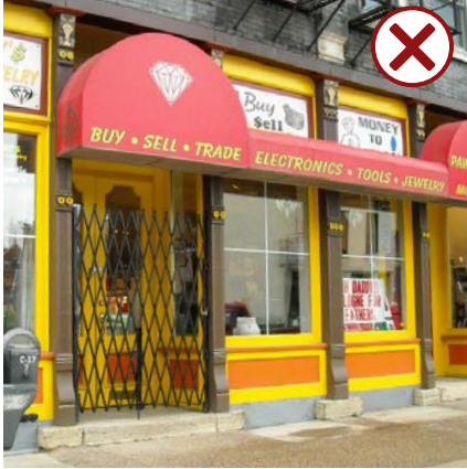
Do not install curved form awnings on a rectangular opening or use colors that are not compatible with the structure.
