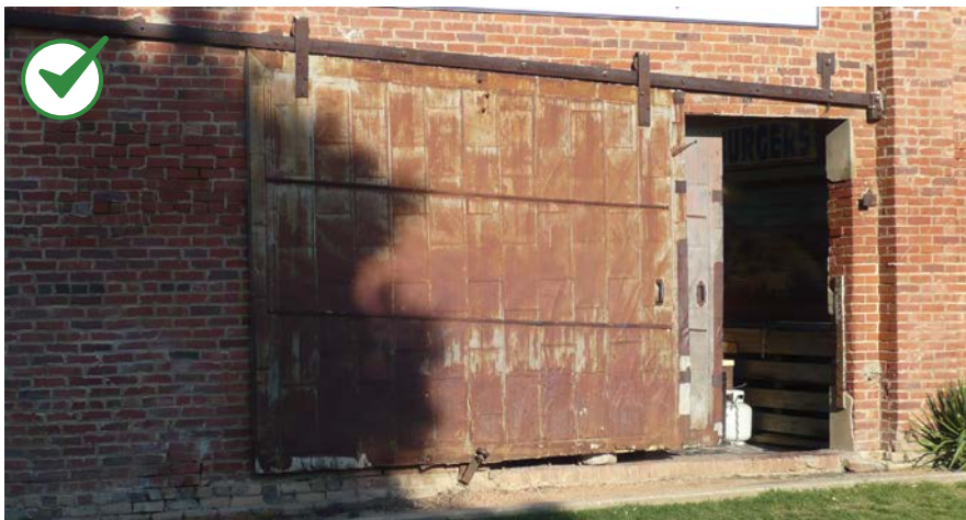
Preserve historic doors and their openings.
