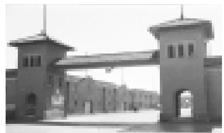
The entrance to the Horse and Mule Barns is marked by two two-story towers, each with round arched openings at the base and three small round arched openings on the second level.
