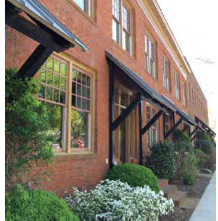
Use a consistent plant palette throughout the property.
