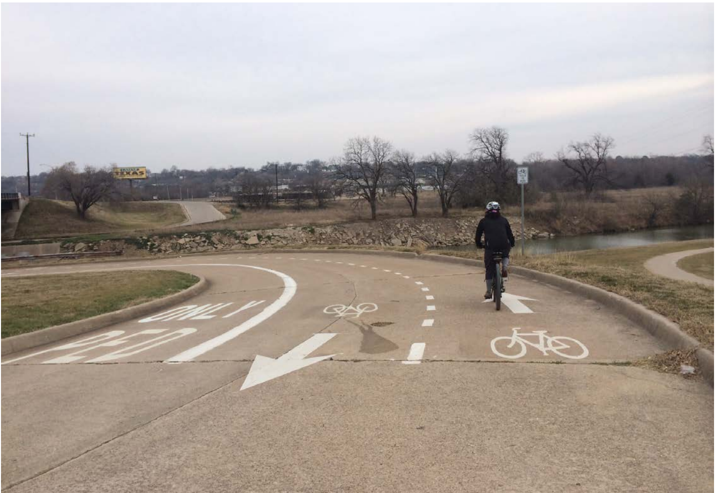
The ATP lays out a vision for comfortable and connected walking and bicycling facilities such as these on University Drive and Trinity River Trail. (Photo credit: City of Fort Worth)
