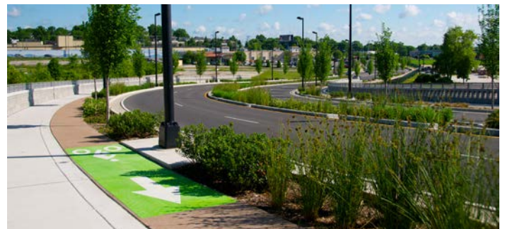
Figure 29. Sidewalk-level Separated Bike Lane (Photo credit: Toole Design)
