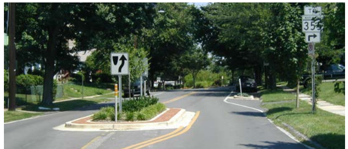
Figure 36. This island in Maryland narrows the travel lanes and creates a curve in the road, both of which cause vehicles to slow down (Photo credit: Toole Design)
