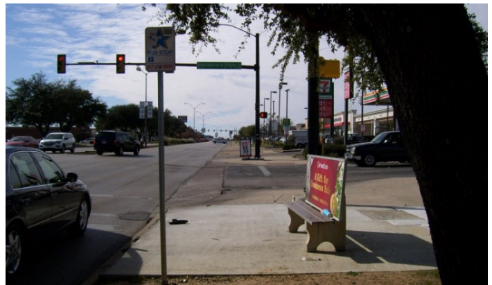
Figure 49. Bus stop landing pad (Photo credit: Trinity Metro)
