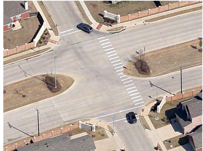
CROSSWALK ON A HIGH-SPEED ARTERIAL
