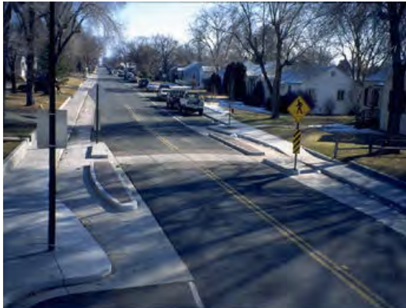
EXAMPLE OF A TRAFFIC CALMING SIDEWALK EXTENSION
