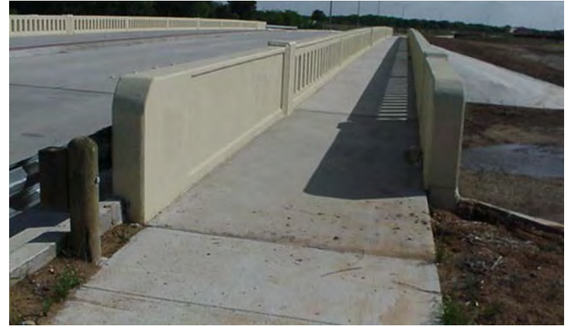
BRIDGE OVER ELIZABETH CREEK IN FAR NORTH FORT WORTH
