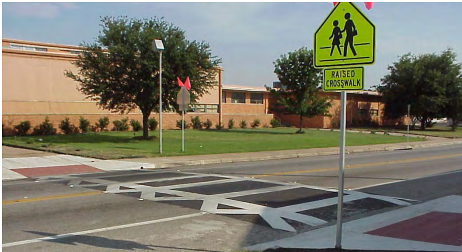
RAISED RIGHT TURN PEDESTRIAN CROSSING. PHOTO CREDIT: DAN BURDEN
