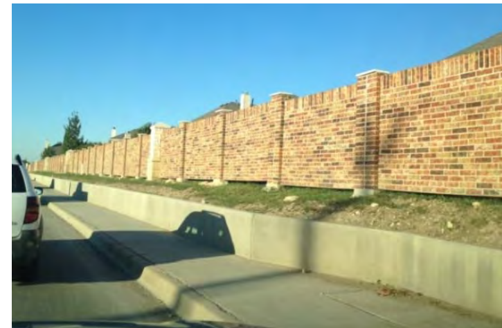
SIDEWALK ON NEWLY CONSTRUCTED ARTERIAL IN FORT WORTH WITHOUT A BUFFER ZONE
