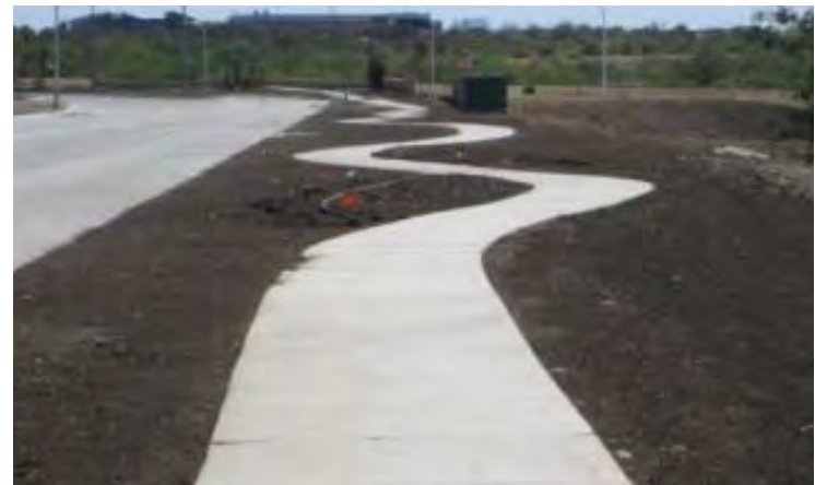
MEANDERING SIDEWALK ALONG A NEW FORT WORTH ARTERIAL
