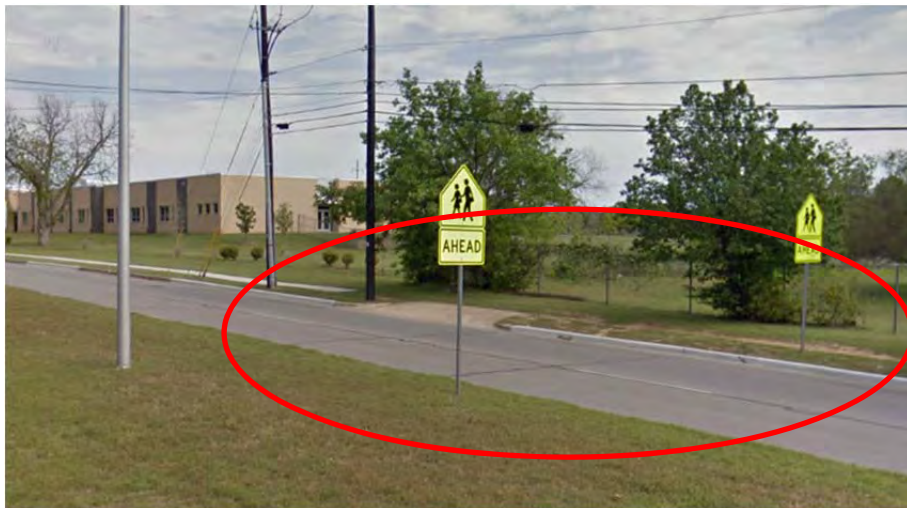
JOHN T WHITE SCHOOL - LACK OF CONTINUOUS SIDEWALKS
