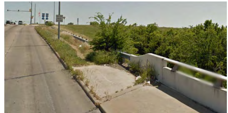
DESIRE LINES ON EASTCHASE PARKWAY
