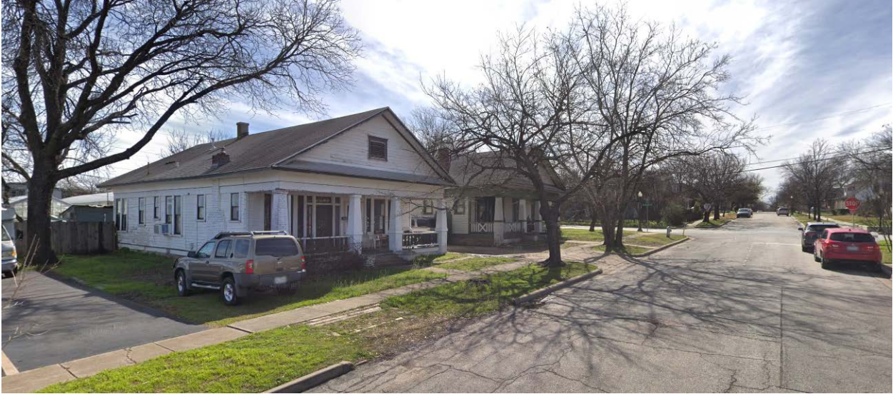
Figure 5. View looking south east, along 5 th Avenue, just north of W Allen Avenue
