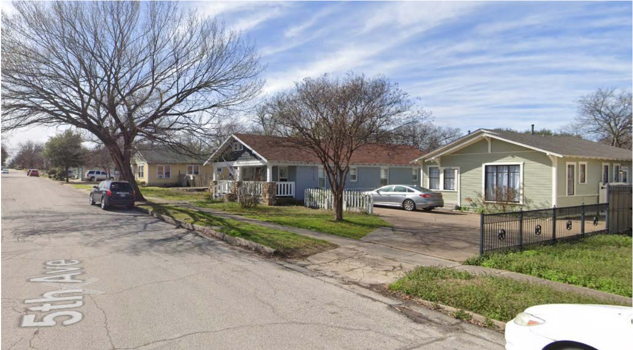
Figure 3. View of immediate context as seen from 5 th Avenue, looking south west
