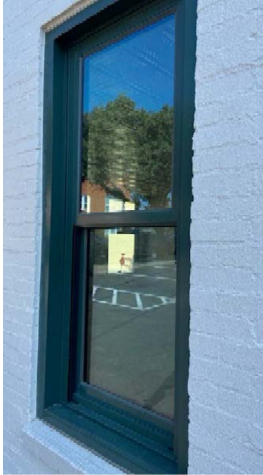
Fig. 10 – Showing detail of compatible new window.
