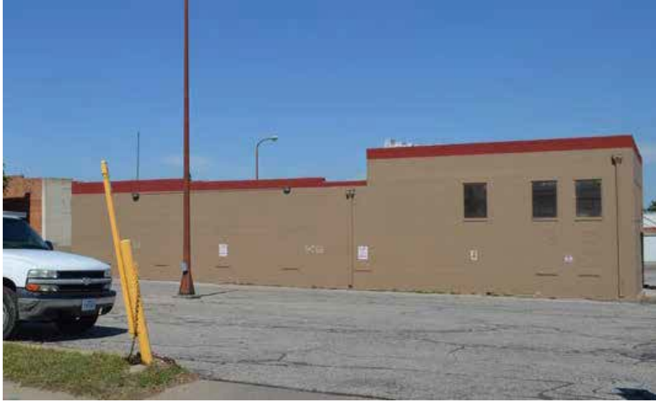
Fig. 4 – West façade prior to rehabilitation. Note that many original window openings had been enclosed.
