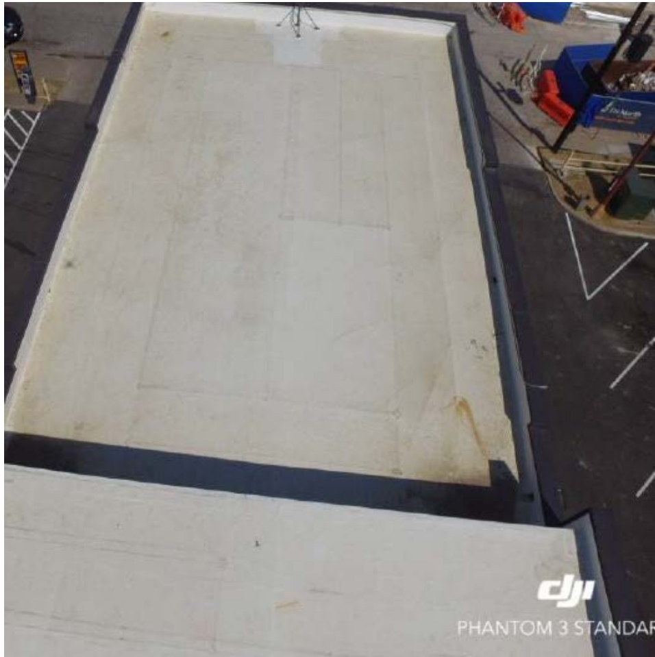
Fig. 8 – Showing new TPO roof system and parapet caps.
