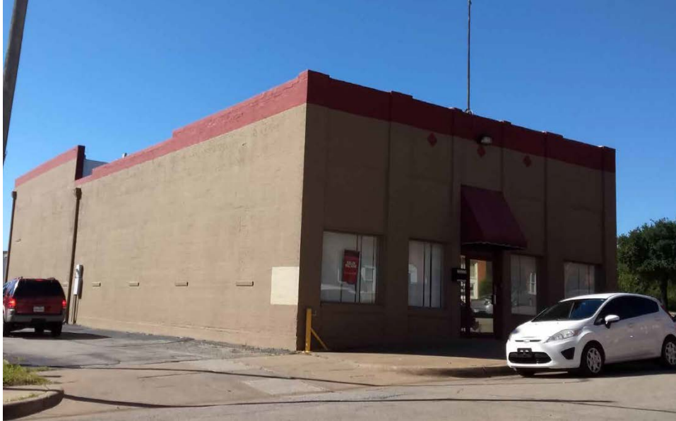
Fig. 2 – Main structure prior to rehabilitation.
