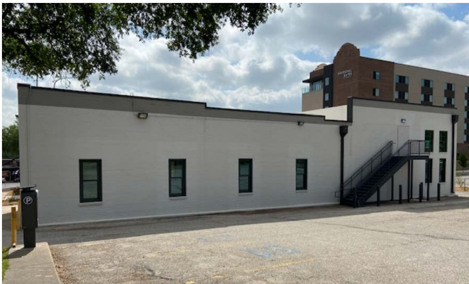
Fig. 5 – Showing west façade after rehabilitation, including reinstated windows in original openings.
