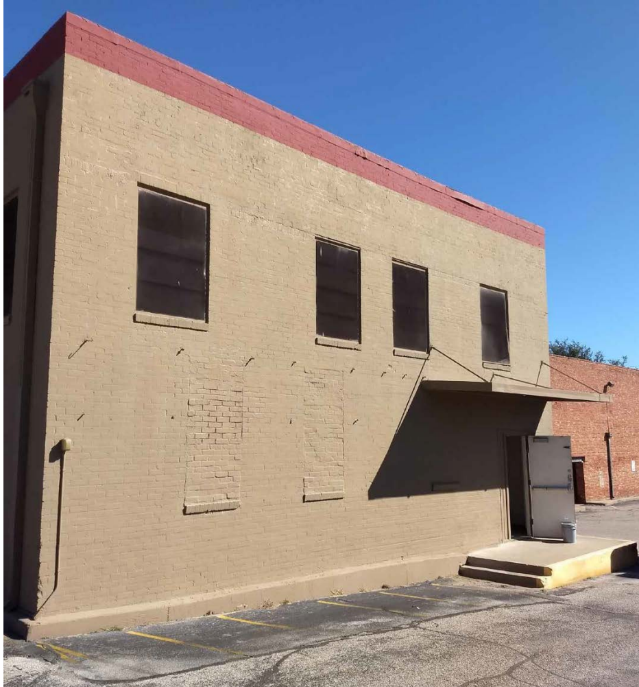
Fig. 6 – Showing rear elevation prior to rehabilitation. Note enclosed window openings and damaged parapet cap. Windows in existing second story opening were used to inform the design of compatible window replacements in bricked-in window openings.
