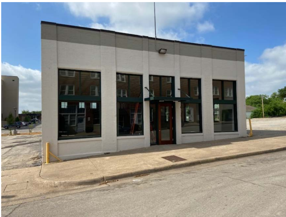
Fig. 3 – Front façade after rehabilitation. Note new paint, reinstated storefront and windows, compatible entrance canopy, and compatible new front doors.
