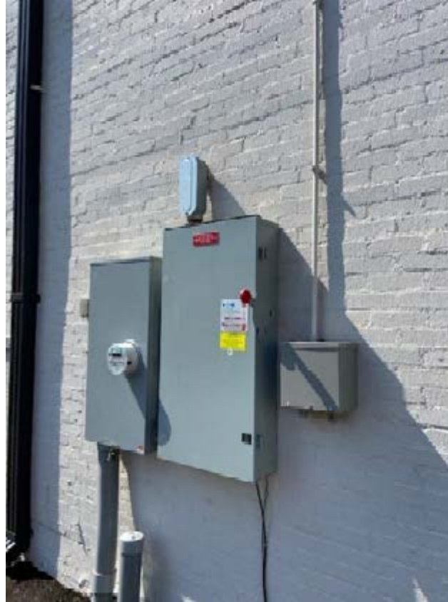
Fig. 9 – Showing new electrical panel as part of MEP system upgrade.
