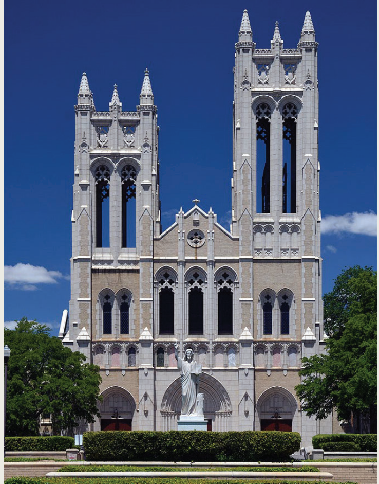
Figure 3-64. Photograph of the extant First Methodist Church at 800 W. 5th Street, constructed in 1930. Source: Fort Worth Architecture, accessed September 17, 2019, http://www.fortwortharchitecture.com/fumc.htm .
