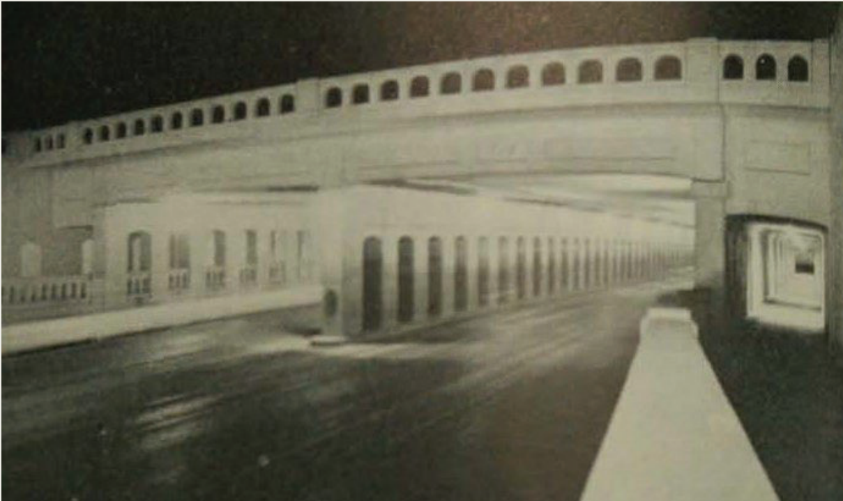
Figure 3-29. Photo of the Jennings Avenue underpass, ca. 1931. The underpass is extant and is a contributing structure to the National Register-listed Jennings-Vickery Historic District. Source: Kline, Jennings-Vickery Historic District, citing Five Years of Progress: A Final Report of the Five-Year Work Program of the Fort Worth Chamber of Commerce and a Pictorial Record of Growth and Development of Fort Worth in the Last Five Years, 1928-1932 (Fort Worth Chamber of Commerce, 1932), courtesy of the Fort Worth Library.
