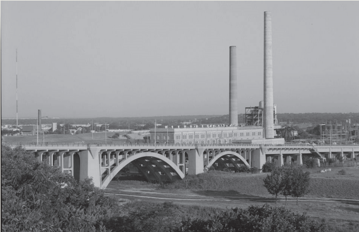
Figure 3-26. The 1914 Paddock Viaduct, spanning the Trinity River, was designed by engineer S.W. Bowen from the firm of Brenneke and Fay. The extant bridge is listed in the National Register. Source: Joseph E.B. Elliott [photographer], 3/4 View from SE, Main Street Viaduct, Spanning Trinity River at Main Street, Fort Worth, Tarrant County, TX, from LOC, http://hdl.loc.gov/loc.pnp/hhh.tx0777/photos.366621p .
