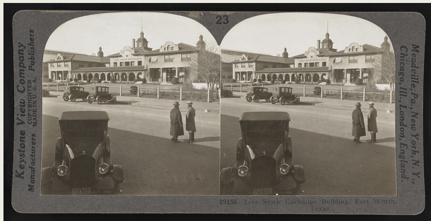
Figure 3-11. Stereographic photo looking toward the livestock exchange, ca. 1928. The building is extant and contributes to the local and NR-listed Fort Worth Stockyards Historic District. Source: Keystone View Company, Livestock exchange Building, Fort Worth, Texas [Photograph] (Meadville, Pa.: Keystone View Company, ca. 1928), from the LOC, https://www.loc.gov/item/93517290/ .
