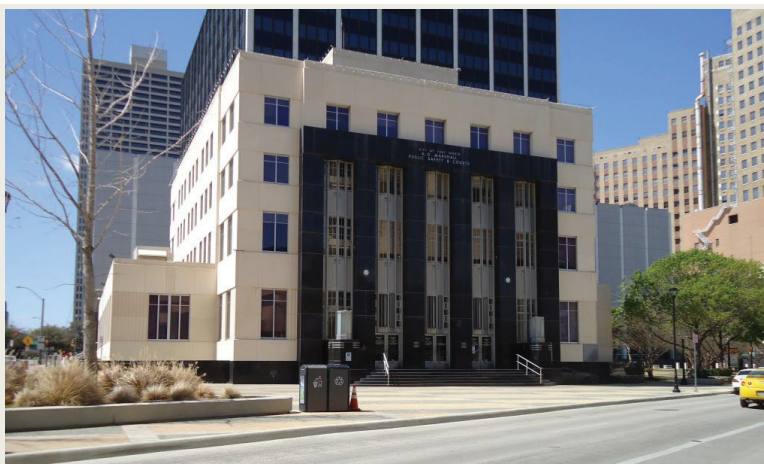
Figure 3-55. Photo of the New Deal Era City Hall (now the Public Safety and Courts Building), constructed in 1938 at 1000 Throckmorton Street. Source: Susan Kline [photographer], "City Hall (Former) – Fort Worth, Texas," The Living New Deal , accessed September 15, 2019, https://livingnewdeal.org/projects/former-city-hall-fort-worth-tx/ .
