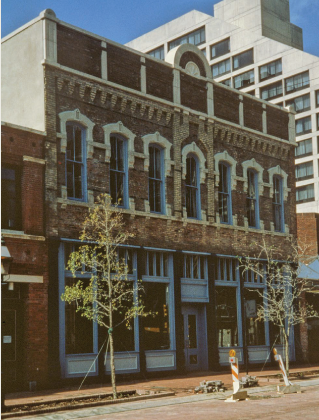
Figure 2-27. View of the ca. 1885 building at 302 Main Street (extant). Source: Source: Historic Fort Worth, accessed August 24, 2021, https://historicfortworth.org/property/bradner-blockweber-building-main/302-main-street/ .
