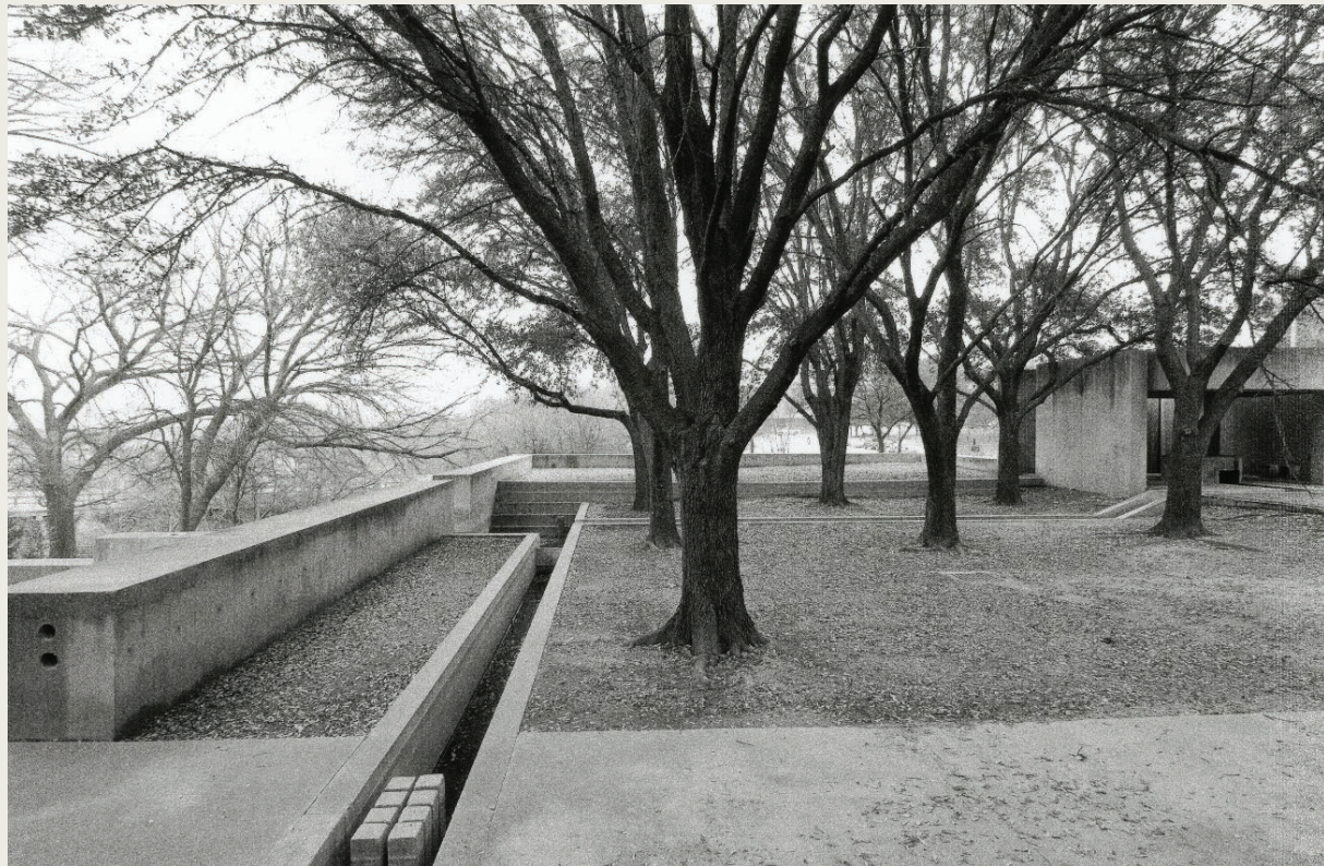
Figure 4-83. Water channel near live oaks in Heritage Park Plaza (looking east), designed by Lawrence Halprin and opened in 1980. The park is listed in the National Register. Source: W. Dwayne Jones and Michal G. Tincup, “Heritage Park Plaza,” National Register of Historic Places Nomination Form, Texas Historical Commission, March 26, 201, 71, from the THC, https://atlas.thc.texas.gov/NR/pdfs/10000253/10000253.pdf .
