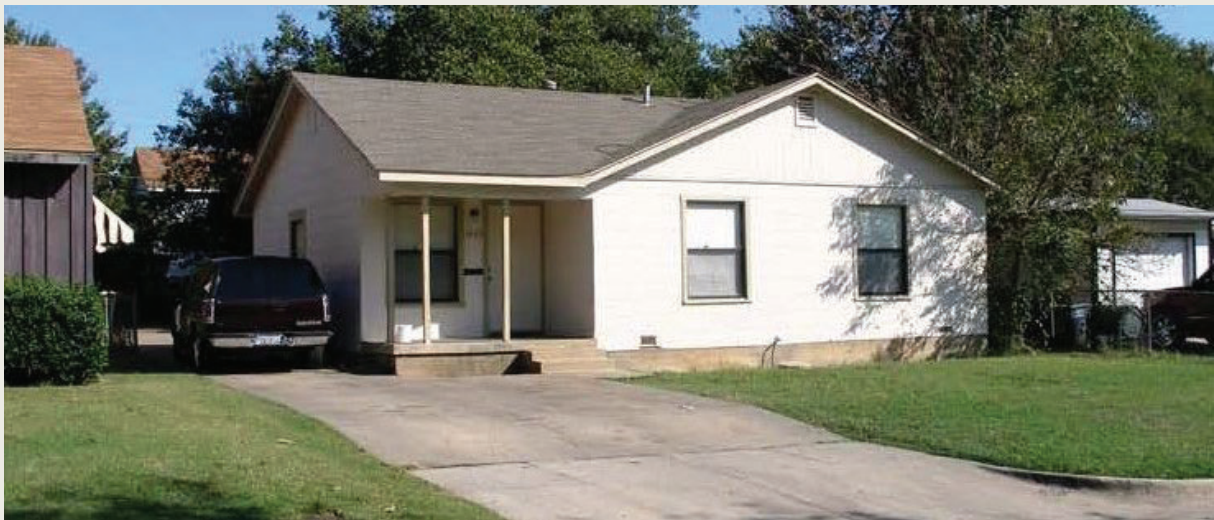
Figure 4-30. An early 1950s Minimal Traditional house at 1229 East Mulkey Street in Morningside. The house is one of several in the 1200 block built in the postwar period. Morningside is a local historic district. Source: Lopez Garcia Group, "Reconnaissance Survey Historic Morningside District, Tarrant County, Texas," 2007, 510.
