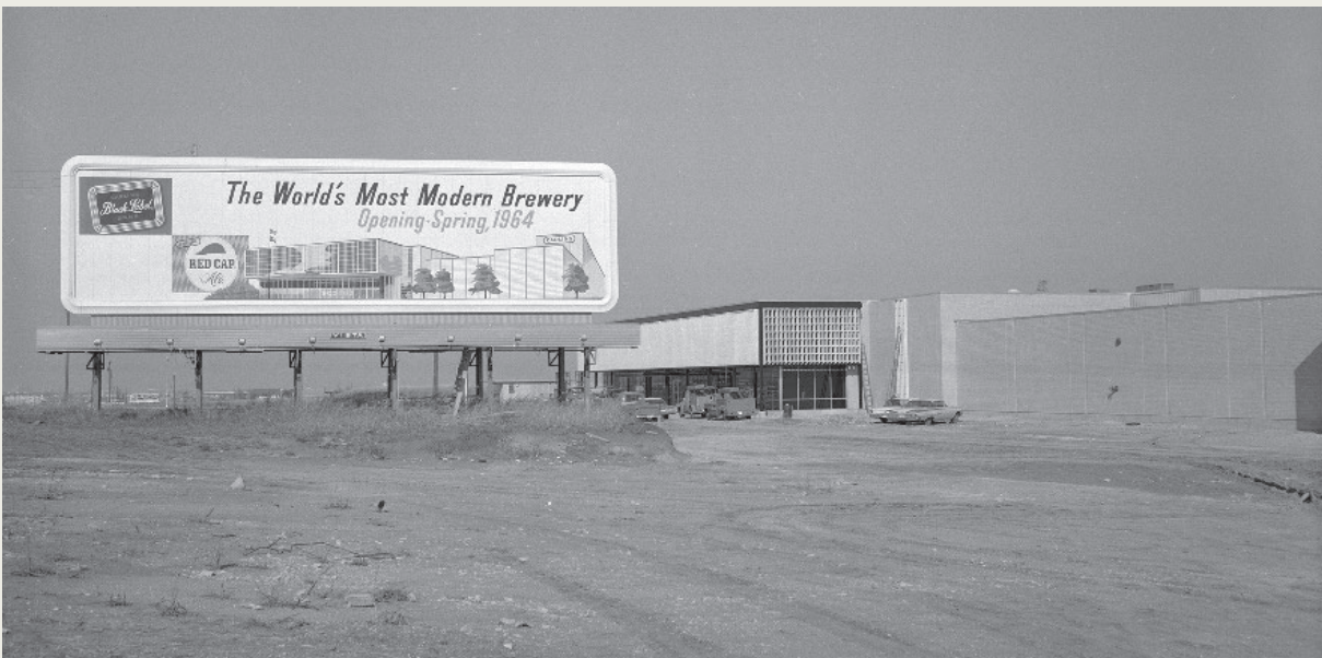
Figure 4-4. The Carling Brewery under construction in Carter Industrial Park, 1963 (extant). Carling occupied the brewery from 1964 to 1966, at which time MillerCoors moved into the building. MillerCoors added an additional 100,000 square feet to the brewery in 1979 and continues operations from the plant. Source: "Carling Brewery, Fort Worth, Texas," Clyde Walton Hill Papers, University of Texas at Arlington Libraries Digital Gallery, 1963, accessed June 9, 2021, https://library.uta.edu/digitalgallery/img/10004717 .
