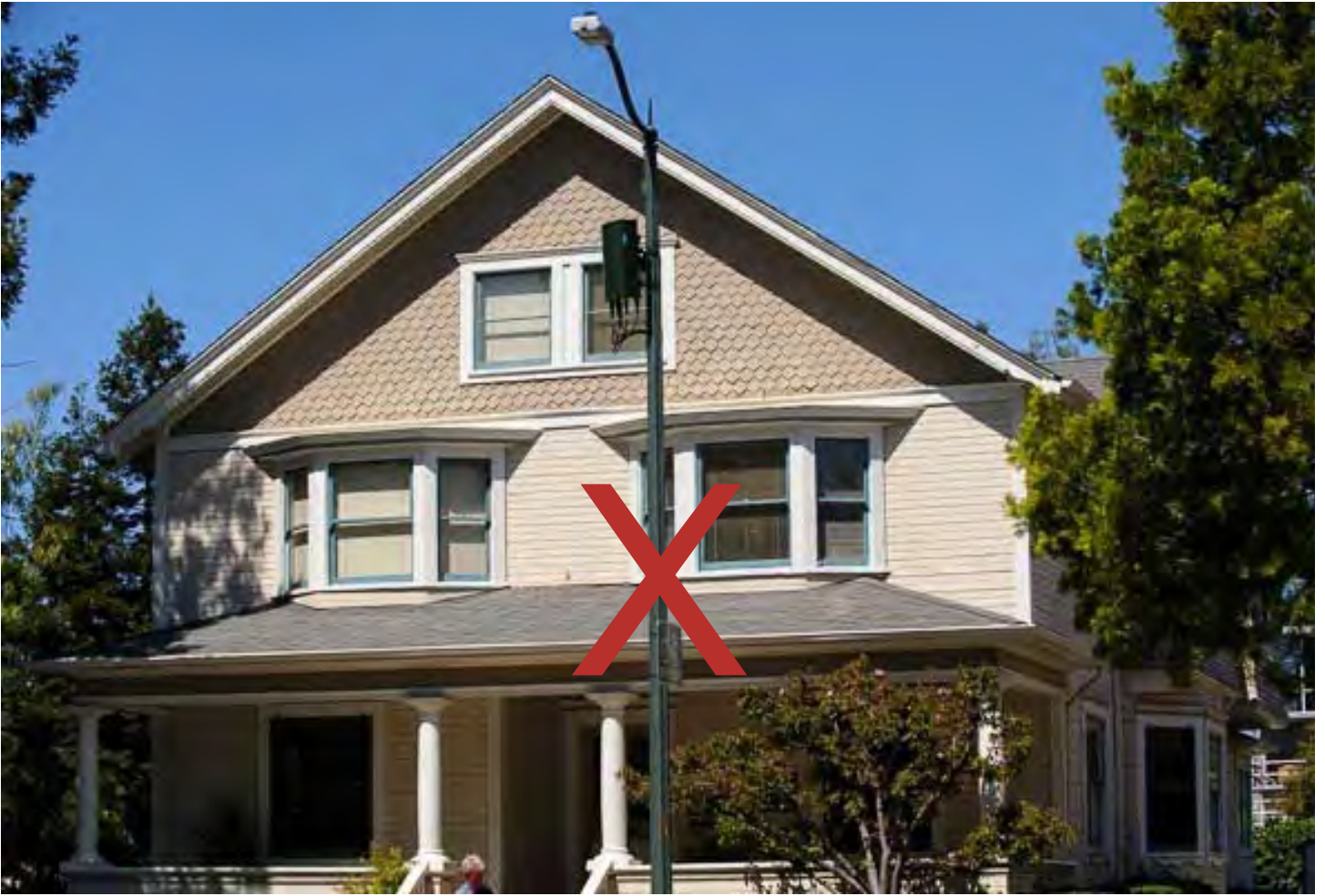
Exhibit 14- The Wireless Facility is located in front of the residential building. Wireless Facilities shall be located where the shared property line intersects the Public Right-of-Way
