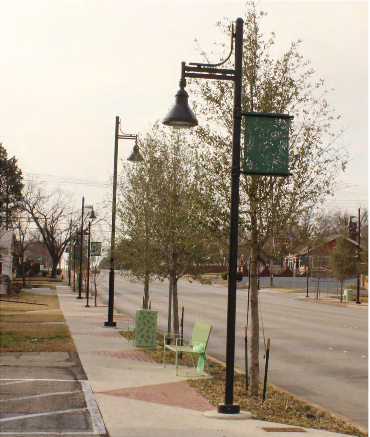
Exhibit 4- Decorative street light with public art. Network Providers shall not install Wireless Facilities on Public Art without written permission from the artist to prevent potential copyright issues.
