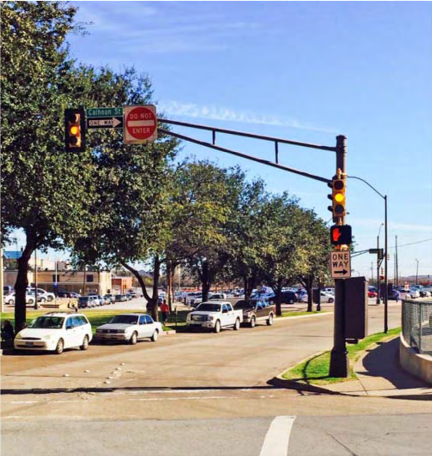
Exhibit 3- Traffic signal structure.
