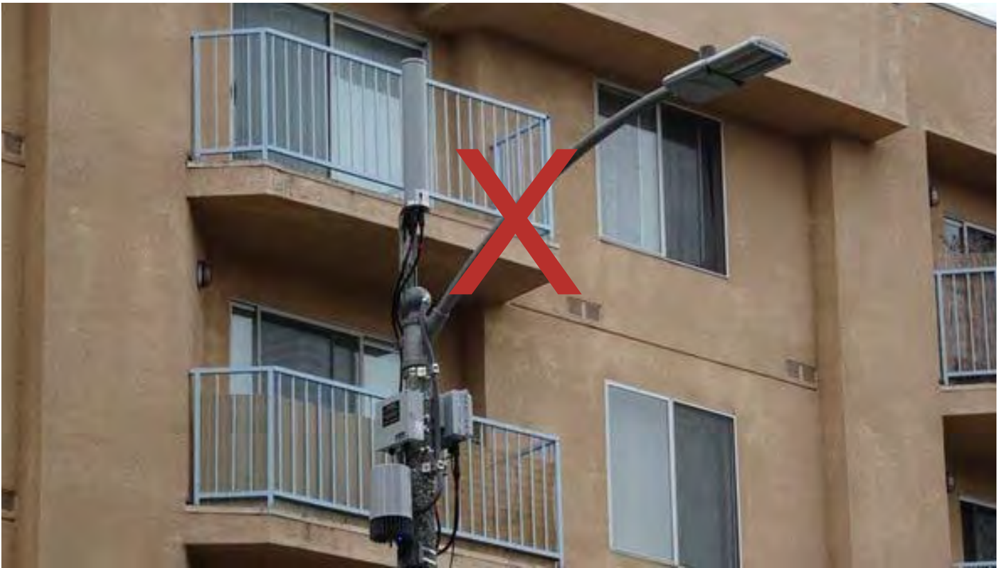
Exhibit 15- Network Node placement shall not impair light, air, or views from adjacent windows.
