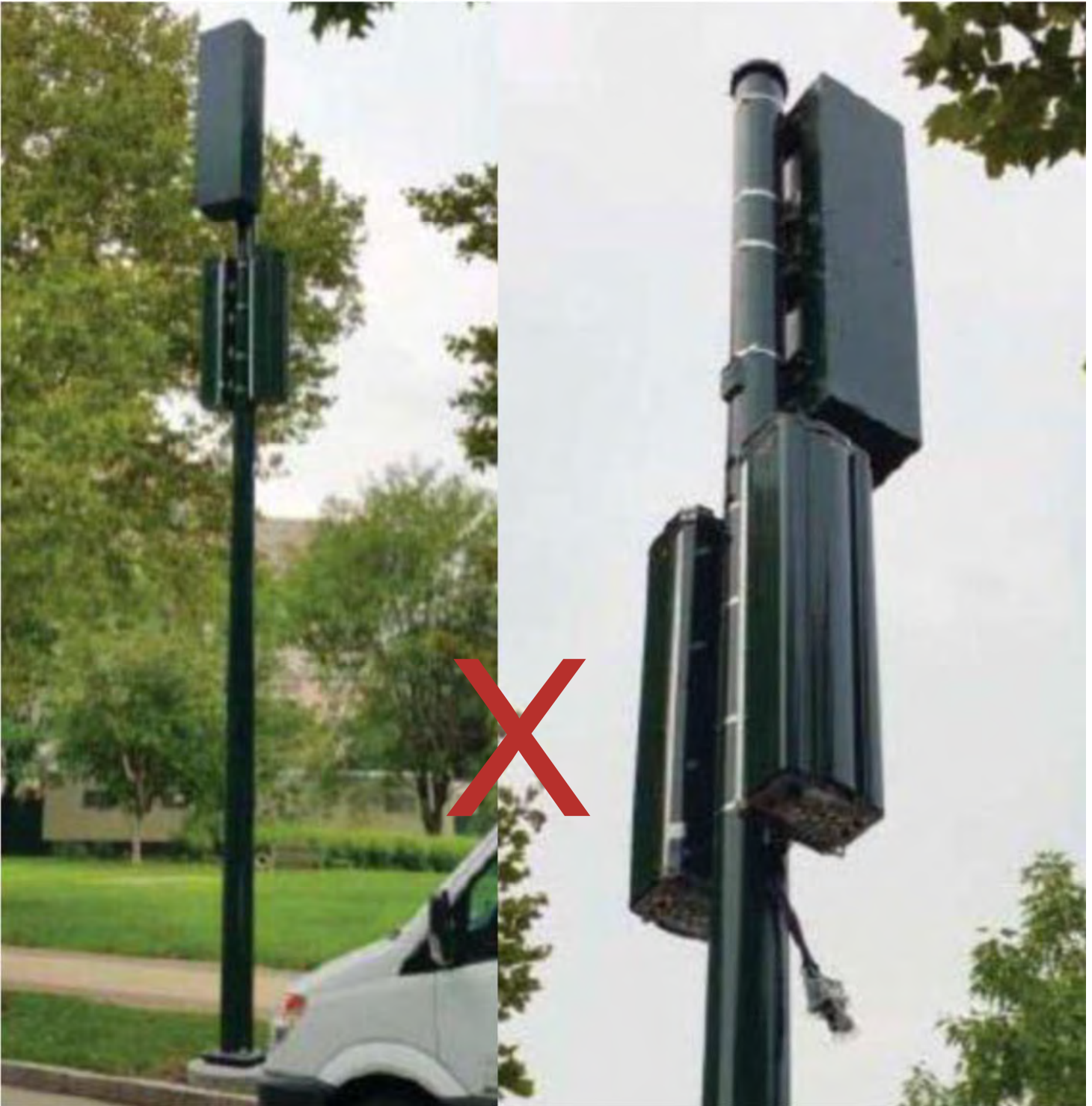
Exhibit 6- In Historic Districts and Design Districts with Decorative Poles more than one Network Node is not allowed because it fails to meet the Concealment standards.
