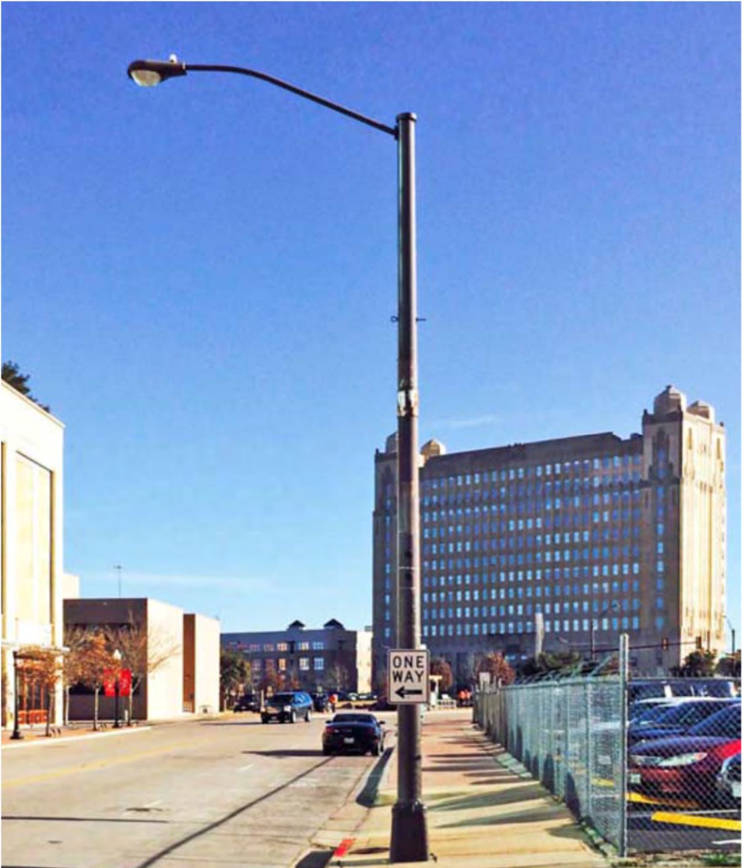
Exhibit 2- Non-decorative streetlights with a height of more than 20 feet.
