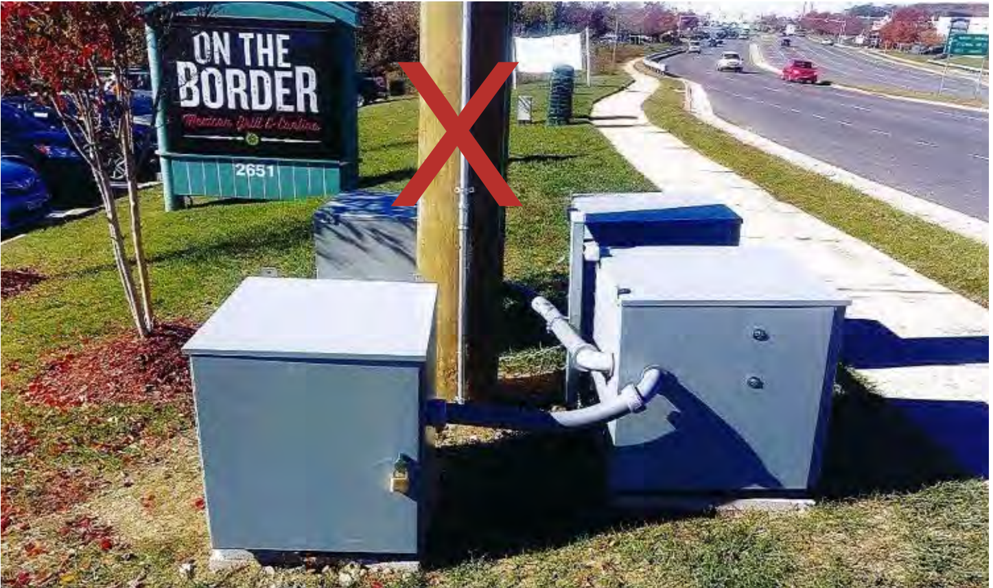
Exhibit 11- Equipment shall not be placed adjacent to the walkway in a manner that diminishes the comfort of pedestrians or be located within the Pedestrian Clear Zone
