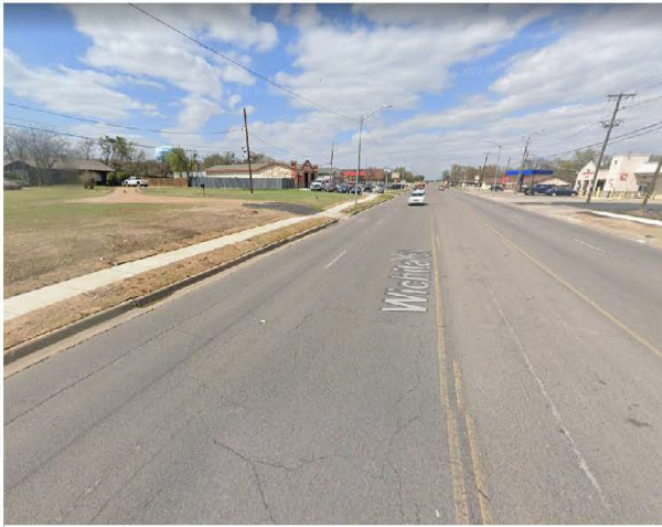
Figure 1-View to the North
