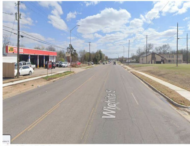
Figure 2-View to the South
