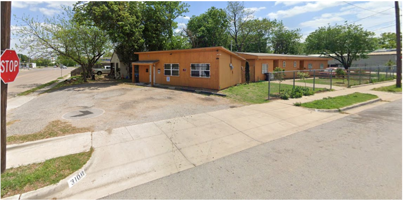
Figure 2- View to the South
