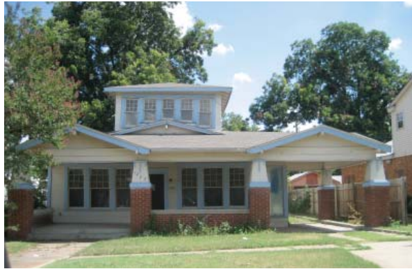
Figure 1. Typical lot condition.
