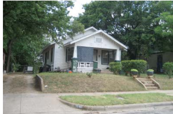
Figure 6. Interior lot condition.
