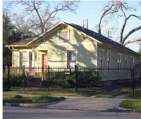
Figure 4.18. Exposed rafter tails and roof overhangs.
