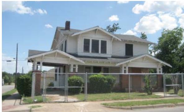
Figure 3. Corner lot condition.
