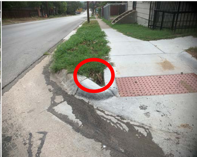
Source: Auditor photograph (Backfilling on 21 st NW and Prospect Ave)
