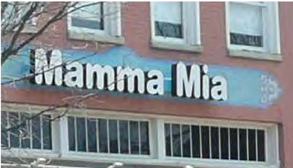
Raceways are discouraged; however when they are necessary they should be painted to match the background. In the above picture the raceway has been painted to match the sign background.
