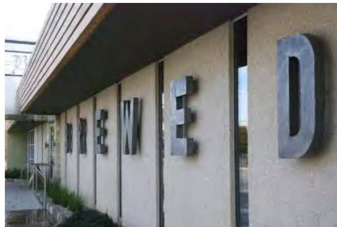
The sign to the left is in keeping with Mid-Century Modern Architecture. Signage should be in keeping with the architectural style of the building.
