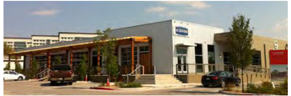
This warehouse space transitions from corrugated metal paneling to stucco.
