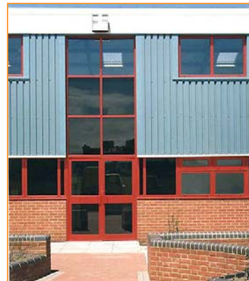
New buildings should have three components; base, middle, and top. Façade articulation is strongly encouraged in terms of wall and window openings and projections, material, and color variations.
