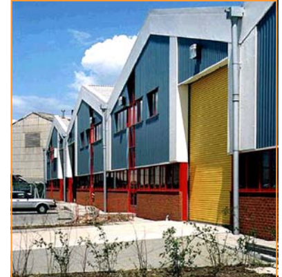
Metal skins used in building facades should blend well with other building materials in terms of color and fenestration.
