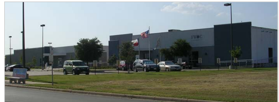
NEZ incentives helped finance the expansion of Tarrant County College's Fort Worth Opportunity Center, a job training facility. The project added 28,129 square feet for new classrooms, laboratory space, and work stations.
