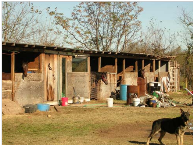
The substandard structure and litter make this location a code violation.
