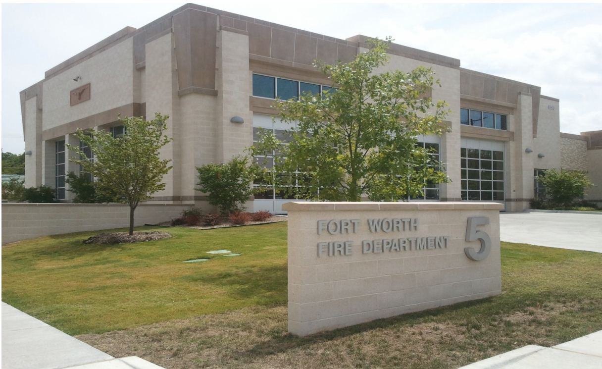
Fire Station #5 - AFTER
