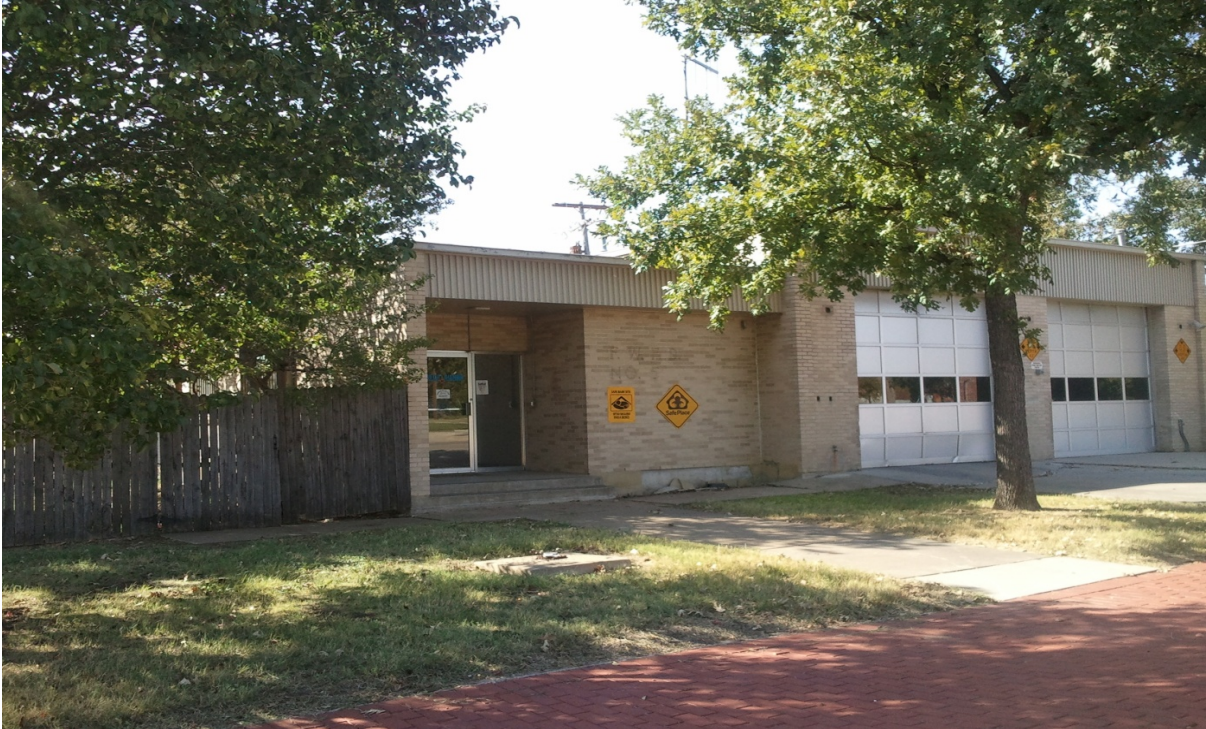
Fire Station #5 - BEFORE
