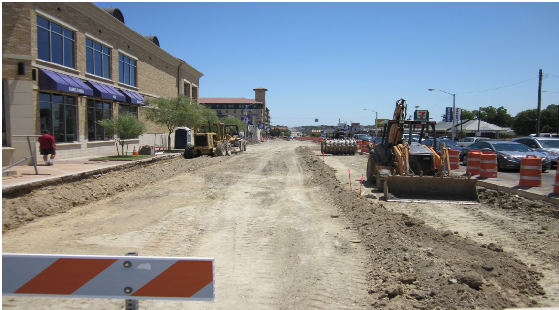
West Berry Reconstruction (Before)
