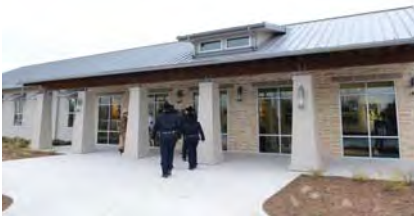
Figure 32: New Mounted Patrol Facility.
