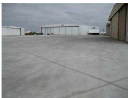
Figure 42: Completed Apron A project at Meacham Airport.
