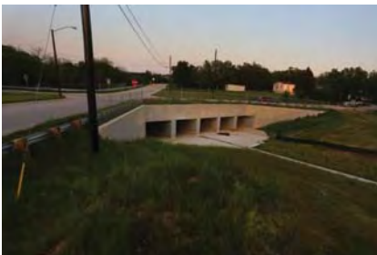
Figure 34: New bridge at the intersection of Butler St. and McClure St. that eliminated a very hazardous low water crossing which was the site of 3 fatalities in 2004.
