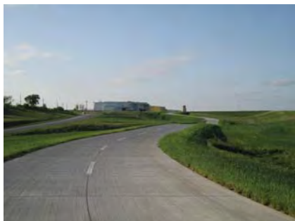
Figure 41: Completed Perimeter Road project at Meacham Airport.
