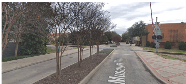
Example of an enhanced crossing in a quiet zone on Museum Way. In order to prevent drivers from deliberately driving around lowered railroad gates in this quiet zone, a median barrier is placed in the center of the roadway.
