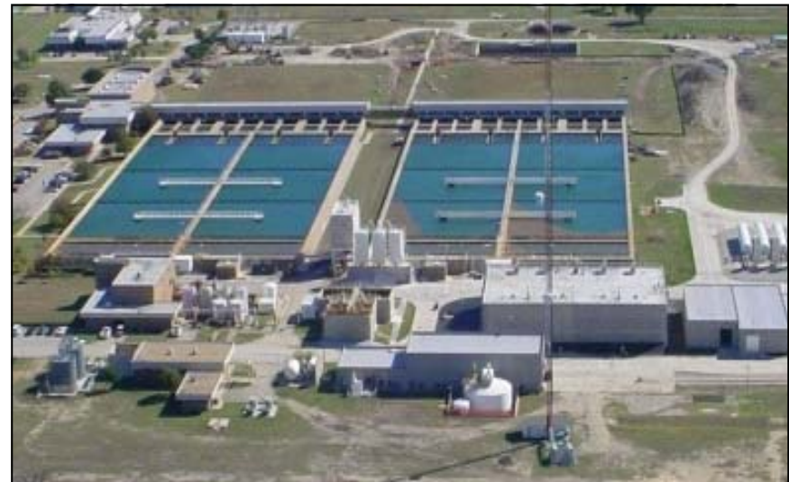
Aerial view of the Rolling Hills Water Treatment Plant and Central Laboratory. The plant was constructed in 1985 and the laboratory was constructed in 1998. Both facilities were funded by revenue from water sales and service charges. (Source: Water Department, 2009.)
