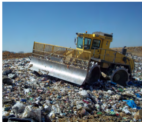
A mechanical compactor being driven at the southeast landfill.
