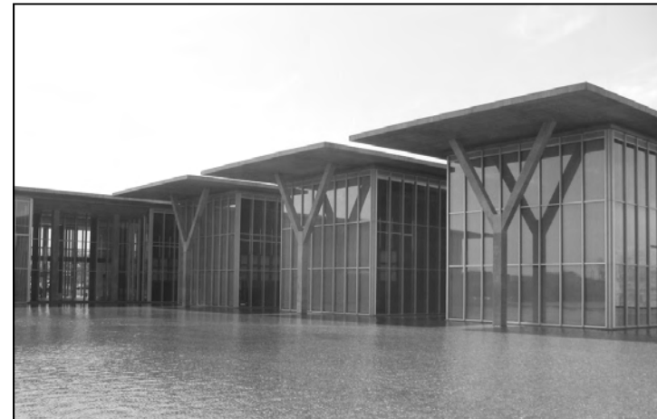
The Modern Art Museum of Fort Worth, designed by acclaimed Japanese architect Tadao Ando, opened in December 2002 in the Cultural District. It embodies the principles of classical Japanese architecture while employing modern Western techniques. The museum features 53,000 square feet of gallery space, a 1.5-acre pond, a cafe overlooking the water, and a 250-seat auditorium. (Source: City of Fort Worth, 2009.)
