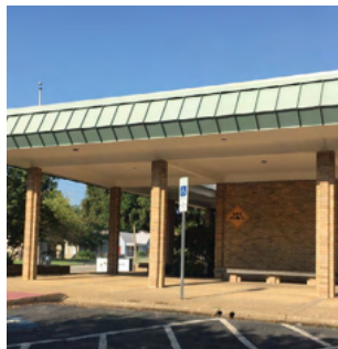
RVS RIVERSIDE 6,300 sf | Built 1967
