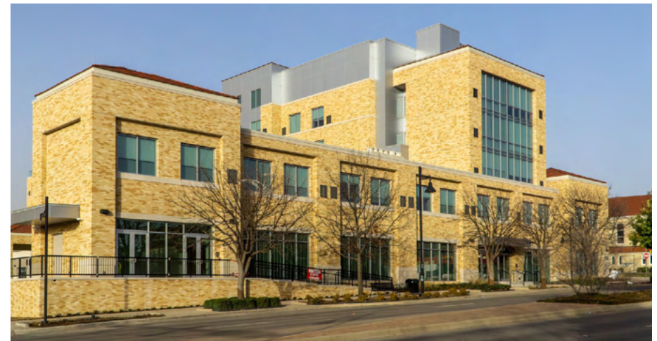
New Hyatt Place Hotel located on Texas Christian University’s campus. (Source: @FortWorthUrban Twitter post, February 2, 2021.)
