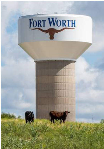
One million gallon elevated water storage tank in Parker County, constructed north of I-20 to serve development in far west Fort Worth.
