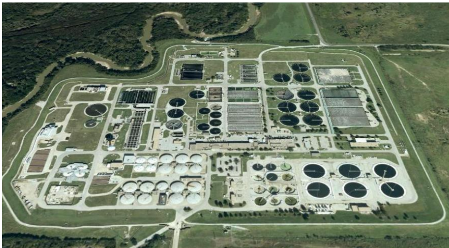
Village Creek Water Reclamation Facility.
