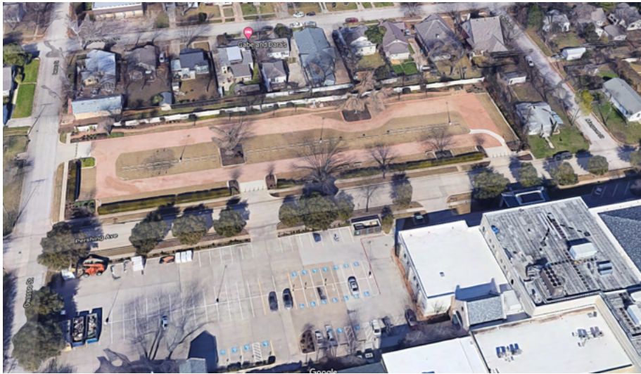
Permeable surface parking lot at Christ Chapel Baptist Church
