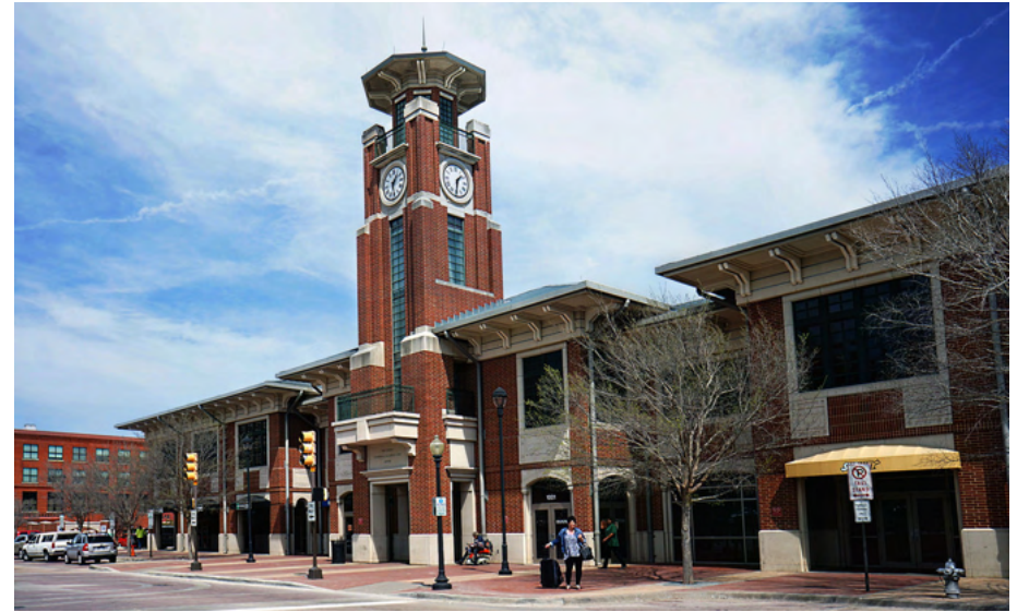
The Fort Worth Central Station, at the intersection of 9th Street and Jones Street in Downtown Fort Worth, exemplifies the value that Fort Worth assigns to mobility. This facility, which opened in January 2002, serves as a terminal for seven transportation modes, including commuter rail services between Fort Worth, Dallas, and the Dallas Fort Worth International Airport. (Source: We Are Dallas Fort Worth Blog, wearedallasfortworth.com )
