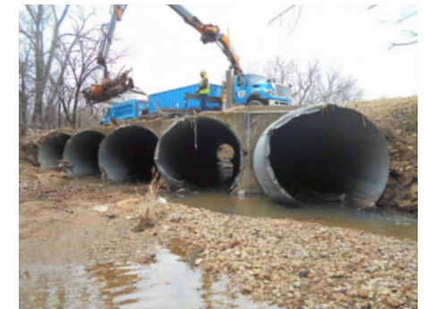
Clearing debris from storm drains.
