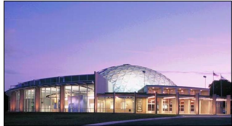
Originally built in 1958, Casa Mañana is a professional theatre landmark in Fort Worth, providing live productions for adults and children. A $4.7 million renovation in 2003 transformed the structure into a 21st-century theater, creating a new 11,400 square foot steel-and-glass lobby to accommodate capacity crowds, and a stage and audience chamber featuring a modified thrust/proscenium stage configuration. The notable geodesic dome roof, designed by architect Buckminster Fuller, remains intact. (Source: Gideon Toal, 2003.)
