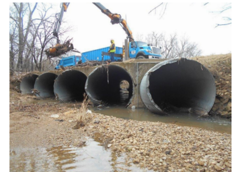
Clearing debris from storm drains.
