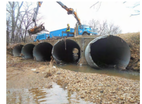
Clearing debris from storm drains.
