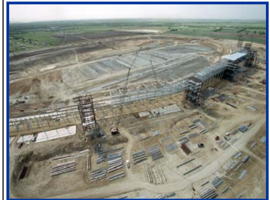
Figure 1.2 Construction of the Texas Motor Speedway grandstands began in 1995.
