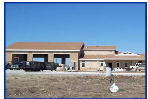
Figure 2.8 Fire Station 11 at SH-114 and Harriet Creek Drive opened in January 2009.
