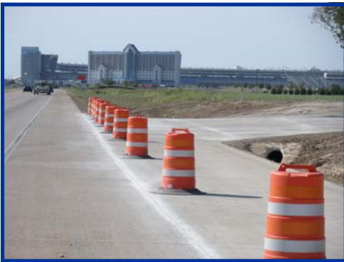
Figure 2.5 Road construction on SH-114 east of TMS
