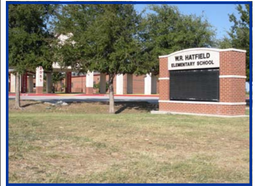
Figure 2.7 Northwest ISD campus includes several schools, athletic facilities, and administration and operations buildings.
