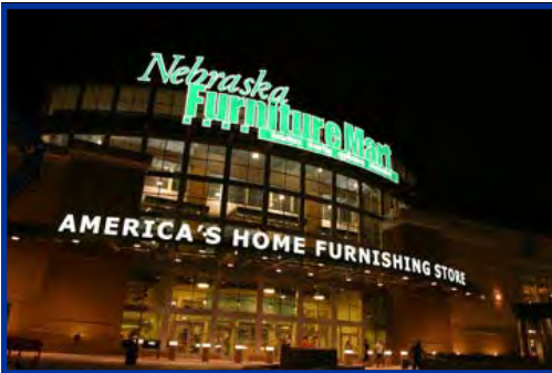
Figure 3.26 Destination retailers such as Nebraska Furniture Mart are adjacent to Kansas Speedway
