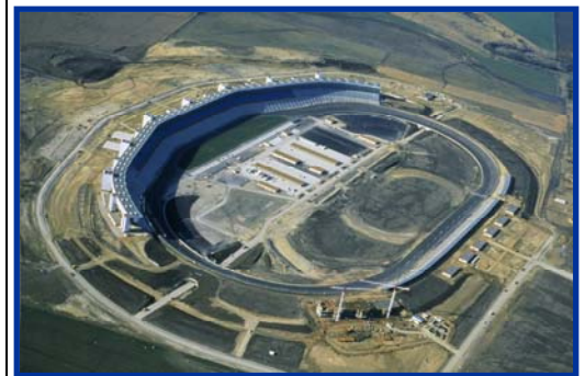
Figure 4.3 Aerial view of TMS during construction.
