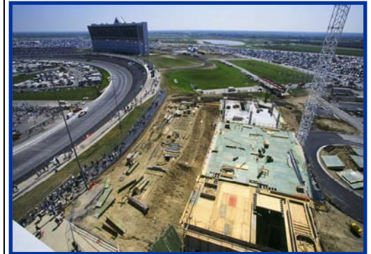
Figure 4.2 Construction of the Speedway Club Tower.
