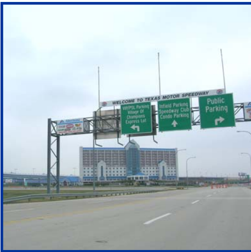
Figure 6.1 TMS has taken steps to improve the efficiency of loading and unloading the parking facility on race days.
