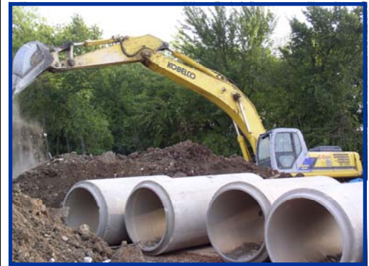
Figure 7.3 Sewer construction in Fort Worth
