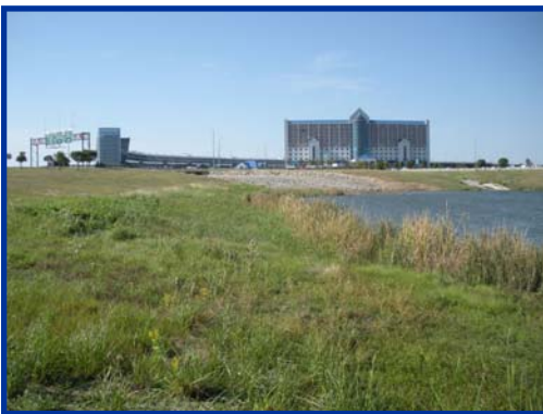
Figure 8.2 The TMS retention pond handles runoff from the southern portion of the site.
