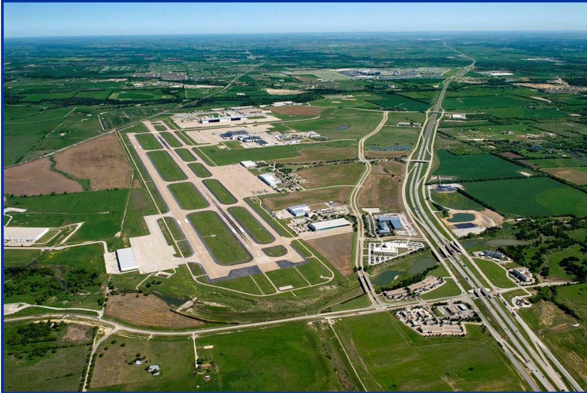
Figure 8.8 Aerial view of Alliance Airport, looking north.
