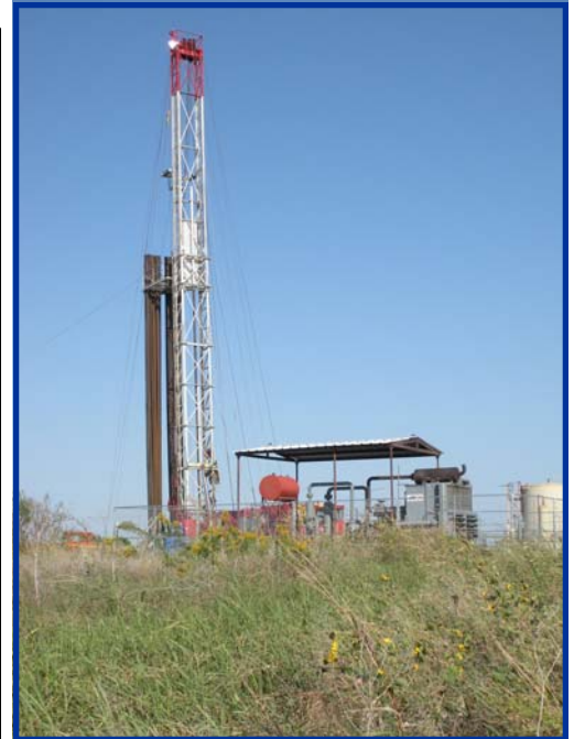
Figure 8.11 Gas well site near TMS.
