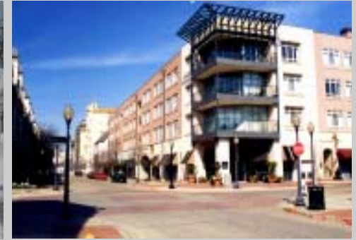
Façade projections and recesses may be dramatic or subtle. This façade combines both approaches.
