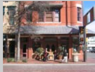
The 20-foot maximum front yard setback encourages an active urban street edge.
