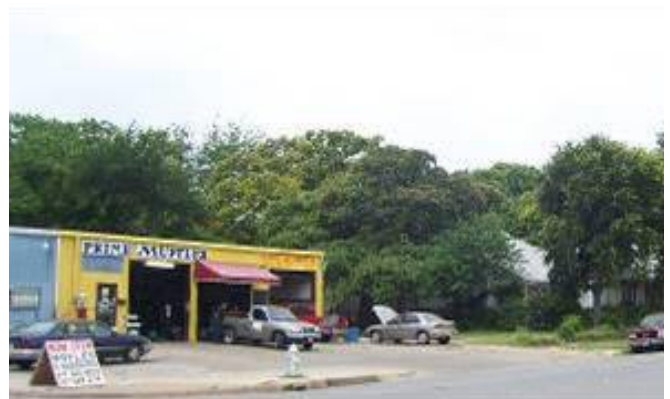
A lack of code enforcement and zoning conflicts present challenges to redevelopment.
