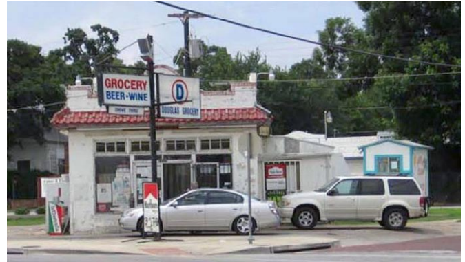
Façade improvements can go a long way towards increasing value.
